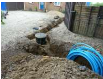
Inspection Chamber 23, Church Road
