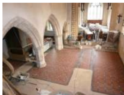
Day eleven Floor tiling and grouting completed
