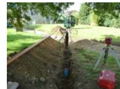
Water and drainage going across the Churchyard
