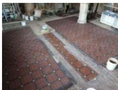
Day ten Tiling complete just the Grouting to finish
