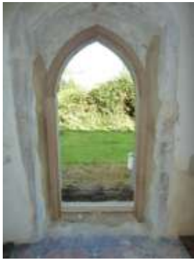
Oak frame in position
