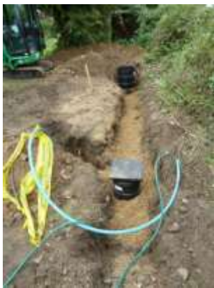
Inspection chamber with branch to the temporary external toilet
