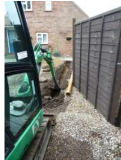
Drainage connected to 23, Church Road
