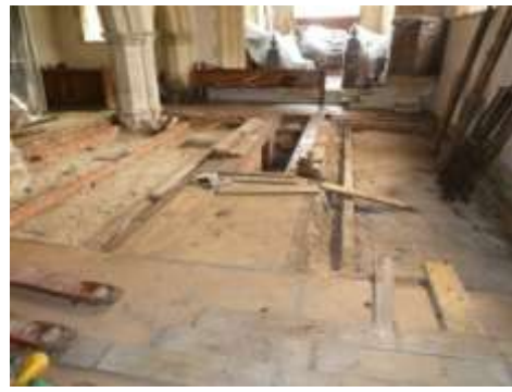
Pews and platforms removed exposing the voids
