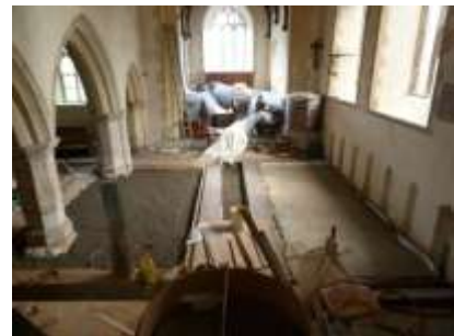
Limecrete slab on right
