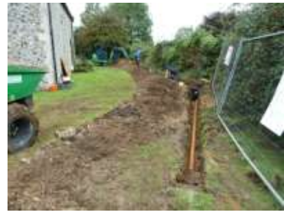
Trench to proposed extension Church kitchen and toilet
