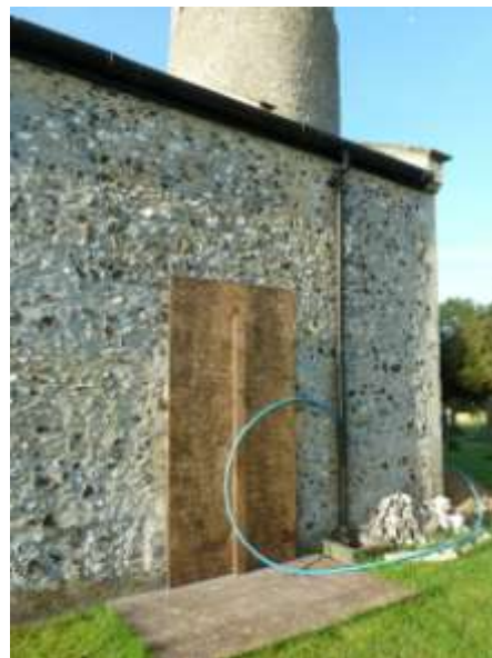
External view of unblocked north door
