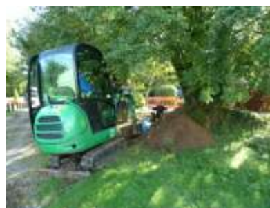
Digging trench through Church boundary
