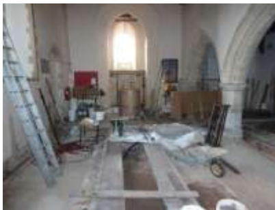
Boiler house and coke store filled with granite chippings
