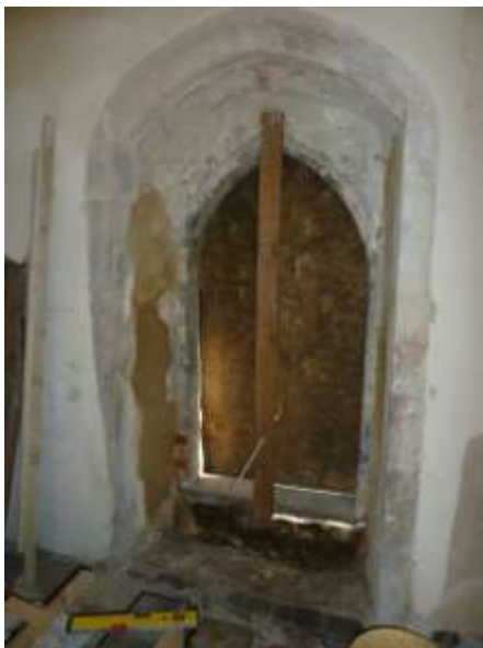
Unblocked north door
