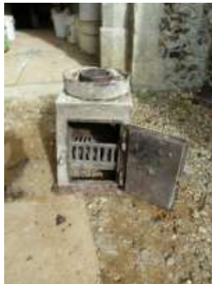
Victorian flue warming stove removed from the vestry
